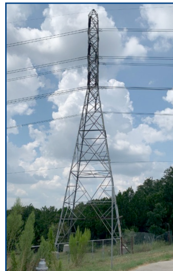
Existing Lattice Structure
